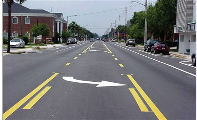
Figure 2. Photo. Three-lane configuration after road diet.
