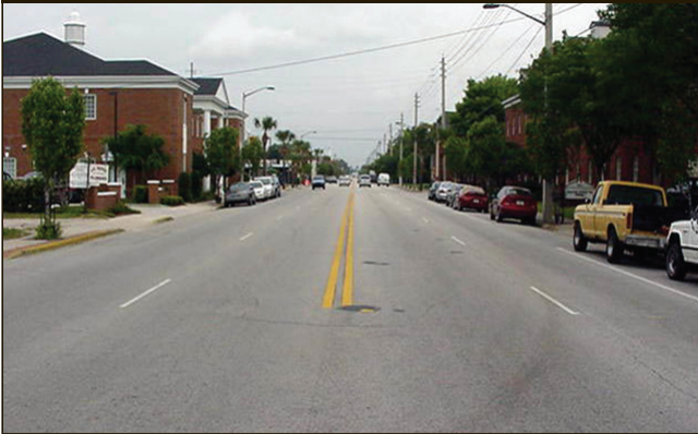
Figure 1. Photo. Four-lane configuration before road diet.
